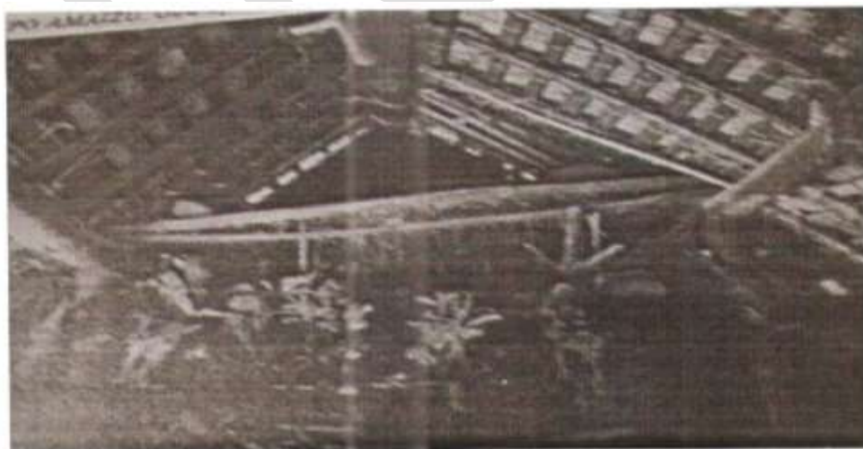
Plate 11; The Space At The Ceiling Level (Attic) Where The Interplay Of Hot And Cool Air Create Cool Interior Of A Residential House. Source: Dmochowski, 1990
