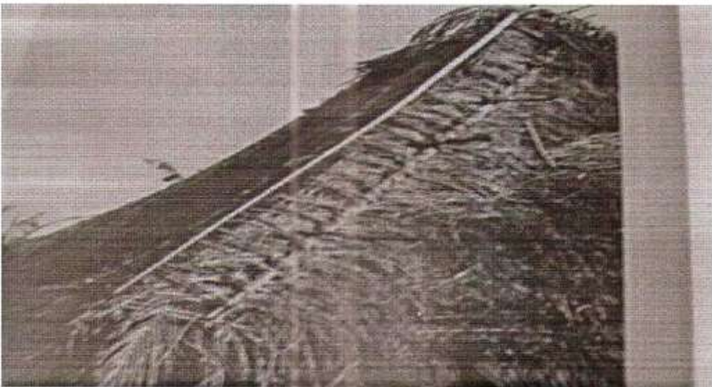
PLATE 13: THE RIDGE COVER (ABUO OTURU) USED TO SECURE THE LONGIVITY OF THE ROOF. SOURCE: DMOCHOSWKI, 1990
