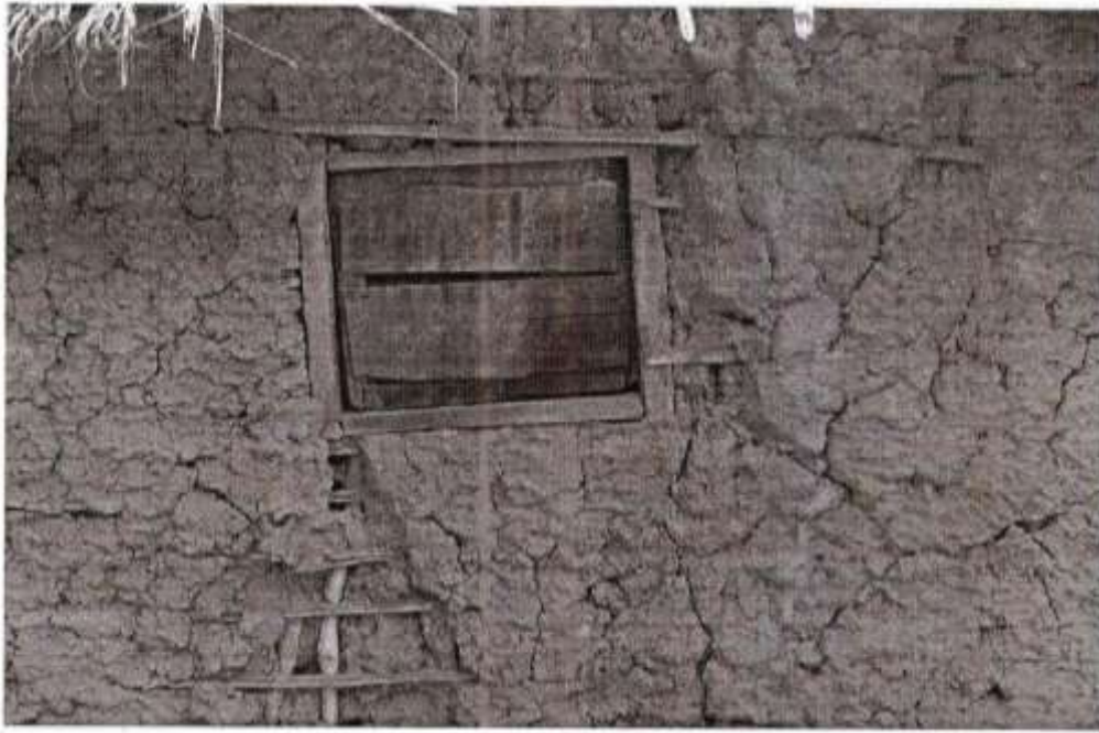
Plate 1: Small Window at The Back (Azoforo Of A Male House At Abam)
